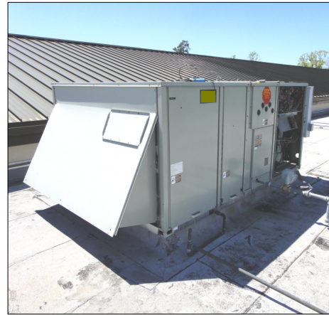
Figure 2a and 2b. New 8½-ton (30 kW) dual-circuit unit installed at Florida test site (left), and retrofitted 20-ton (70 kW) dual-circuit unit at South Carolina test site.
