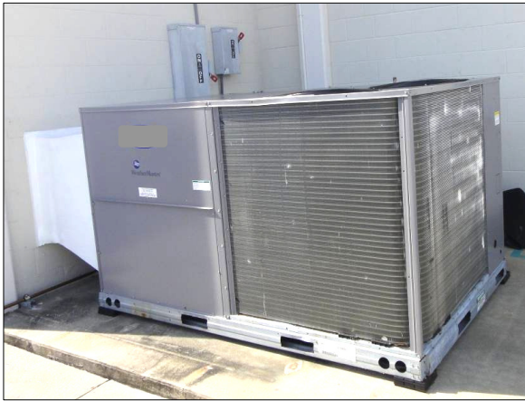
Figure 2a and 2b. New 8½-ton (30 kW) dual-circuit unit installed at Florida test site (left), and retrofitted 20-ton (70 kW) dual-circuit unit at South Carolina test site.
